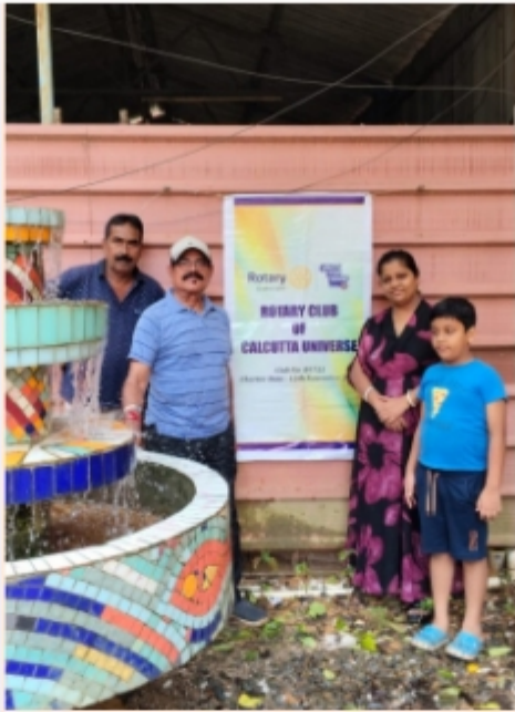
Iron removal Treatment Plant (IRTP) in Housing Complex
